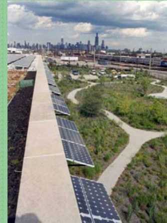
Solar PV installation
